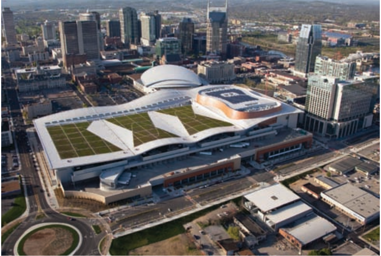
Large solar array on the Music City Center, Nashville, TN.
