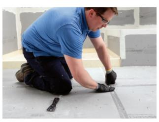
Fasten panels to subfloor with galvanized roofing nails, corrosion-resistant screws or staples.
