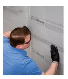
Apply alkali-resistant self-adhesive 2" (51 mm) wide fiberglass mesh tape on all panel seams and corners.
