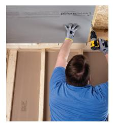
Attach DensShield® Tile Backer with gray side facing outward. Fasten to wood or metal framing with corrosion resistant screws spaced a maximum of 8" (203 mm) o.c. for walls and ceilings. Drive fasteners flush with the gray surface and do not countersink.
