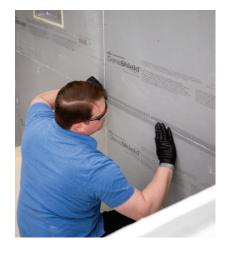
Apply alkali-resistant self-adhesive 2" (51 mm) wide fiberglass mesh tape on all panel seams and corners.
