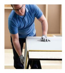
Cut DensShield® Tile Backer using a utility knife to score and then snap, starting with the gray face side. Cuts for penetrations can be made with a jab saw, hole saw or oscillating saw.
