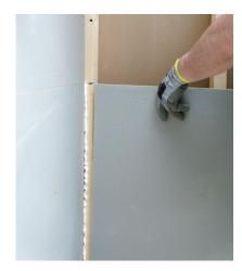
Apply flexible sealant to panel edges before placing adjacent panels. Fit panel edges closely, leaving no gaps between panels. Clean any excess sealant from panel surface after fastening.
