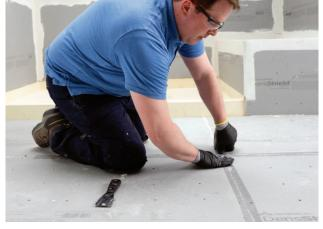
Fasten panels to subfloor with galvanized roofing nails, corrosion-resistant screws or staples.
