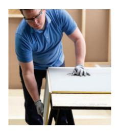
Cut DensShield® Tile Backer using a utility knife to score and then snap, starting with the gray face side. Cuts for penetrations can be made with a jab saw, hole saw or oscillating saw.
