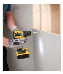
Attach DensShield® Tile Backer with gray side facing outward. Fasten to wood or metal framing with drywall screws or galvanized roofing nails placed a maximum of 8" (203 mm) o.c. for walls and ceilings. Drive fasteners flush with the gray surface and do not countersink. Installed board edges and ends should be butted tightly together.
