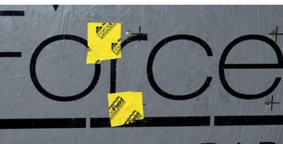
04 OVERDRIVEN FASTENER WITH TAPE TREATMENT
