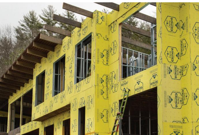
With full control of the products to specify, Chip was not willing to risk using house wrap that would tear or blow off in the high winds and rain. Instead, he knew the right choice for his home was an integrated water-resistant barrier and air barrier (WRB/AB) sheathing system for a building envelope that would keep the elements on the outside.
