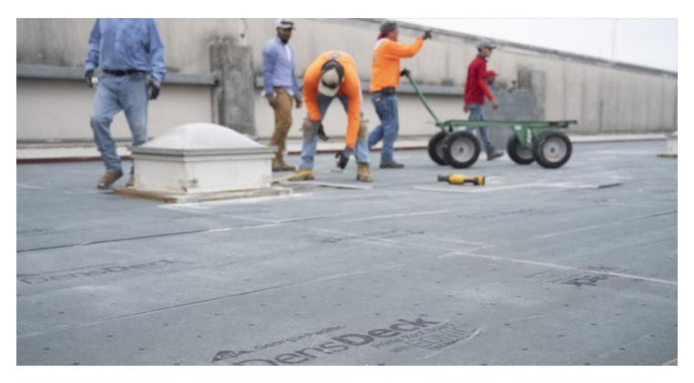
DensDeck® and DensDeck® Prime Roof Boards should not be subjected to abnormal or excessive loads or foot traffic, such as, but not limited to, use on plaza decks or under steel-wheeled equipment that may fracture or damage the panels. Provide suitable roofing system protection when required.
