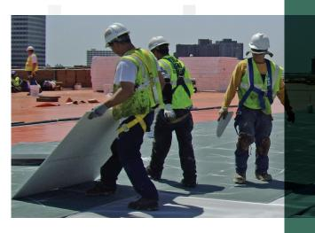
Unfortunately, the reality is that many roofs get wet. And, when exposed to water, cover boards may absorb moisture, resulting in a loss of strength to varying degrees. Consequently, when specifying a cover board, it's important to choose one that offers an enhanced level of performance. According to Downey, this is especially important for owners who are interested in preserving the longevity of their building.
