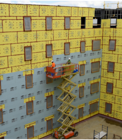
The DensElement® Barrier System installed on Eagle's Landing Apartments, Burlington, Vermont.
