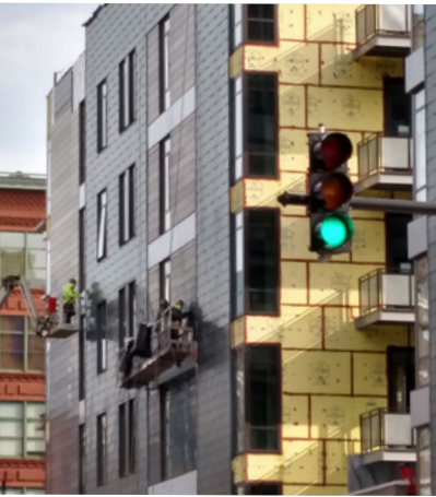
DensElement® Barrier System installation in Chicago, Illinois.
