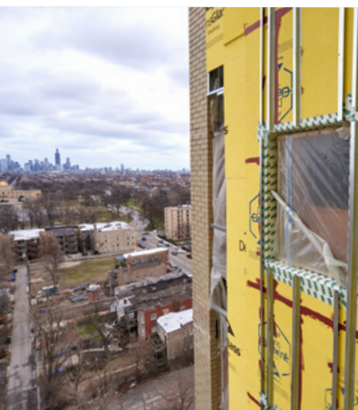
DensElement® Barrier System integrated into wall assembly, Fannie Emanuel, Chicago, Illinois.
